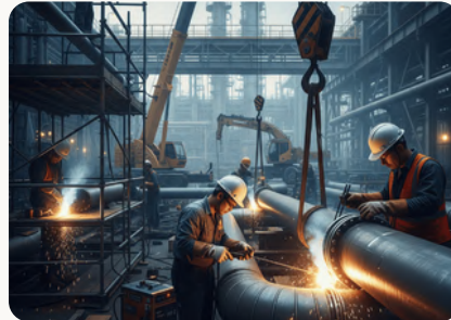
Piping Fabrication and Erection Works
