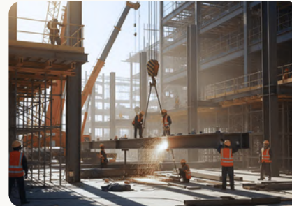
Steel Fabrication and Erection Works
