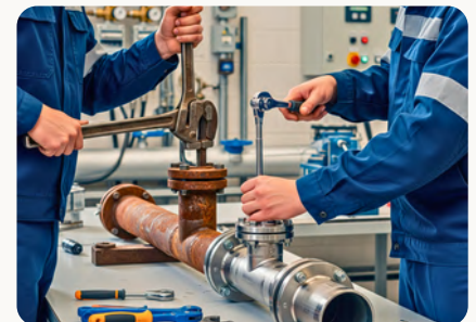
Existing Piping Replacement & Maintenance
