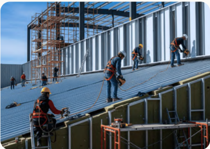
ROOFING AND CLADDING WORKS
